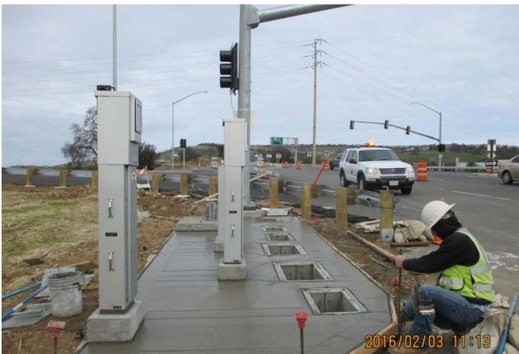
Picture 3 – Traffic signal controllers
