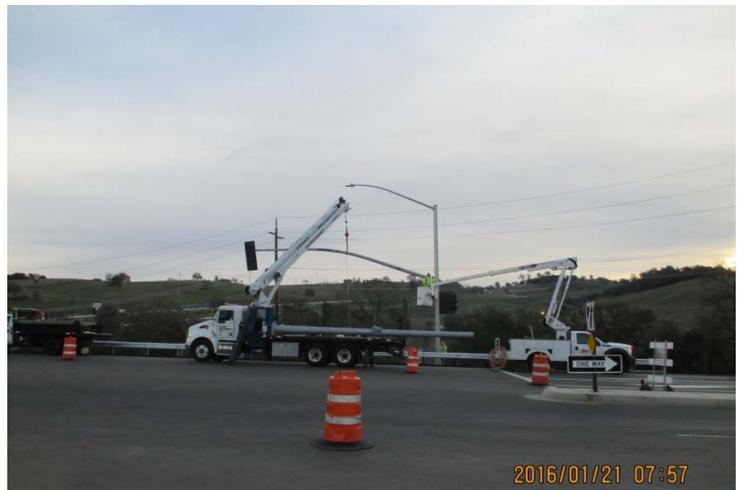
Picture 2 – Installation of traffic signal poles
