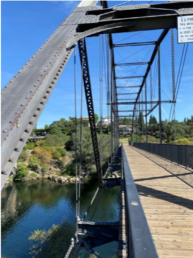
Figure 6: Folsom Historic Truss Bridge with Reduced Deck Width
