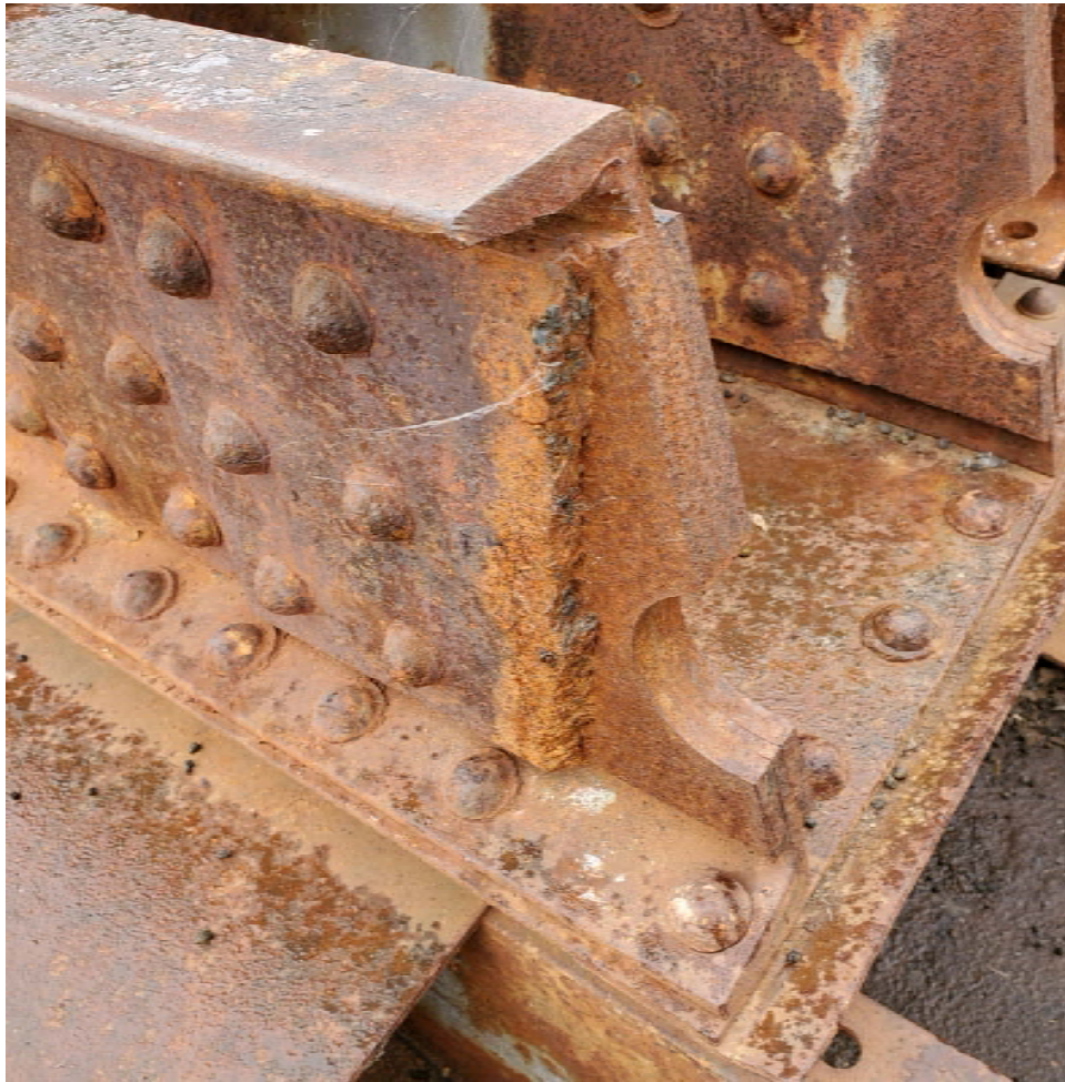
Figure 16: Cut Truss Top Compression Chord Connection Plates
